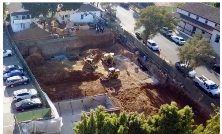
Construction is underway at the new mixed-use development located at 214-226 E. De La Guerra St. With 26 apartments and 5,500 SF office space, The Radius/KIBO Group project is expected to be completed in early 2021.
